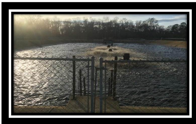
Influent wastewater feeding into the Big Basin for aeration
