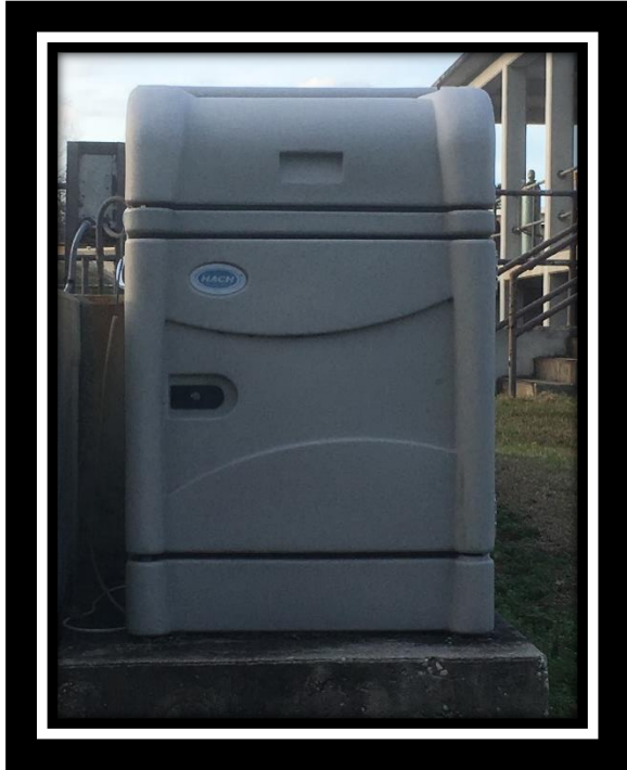
Refrigerated composite sampler is used to collect a 24- hour composite sample on treated effluent for permitted parameter analysis
