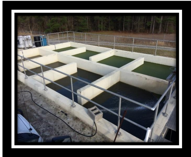
Contact Chamber – Chlorination kills bacteria as wastewater travels through the chambers
