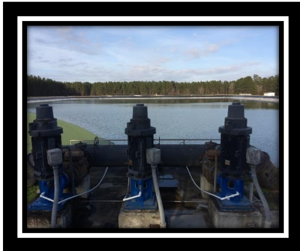
3 – 300 HP pumps that spray treated effluent from the 35 million gallon holding pond onto 637.3 acres
