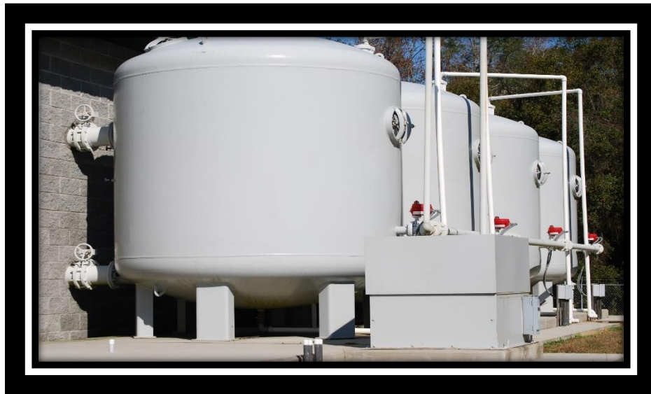
Iron Filtration for removal of iron that occurs naturally in ground water
